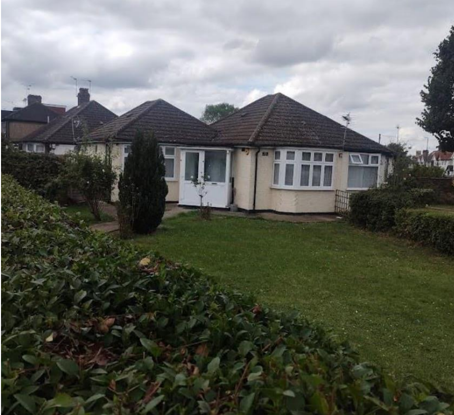
Front Elevation of 40A Somervell Road:
