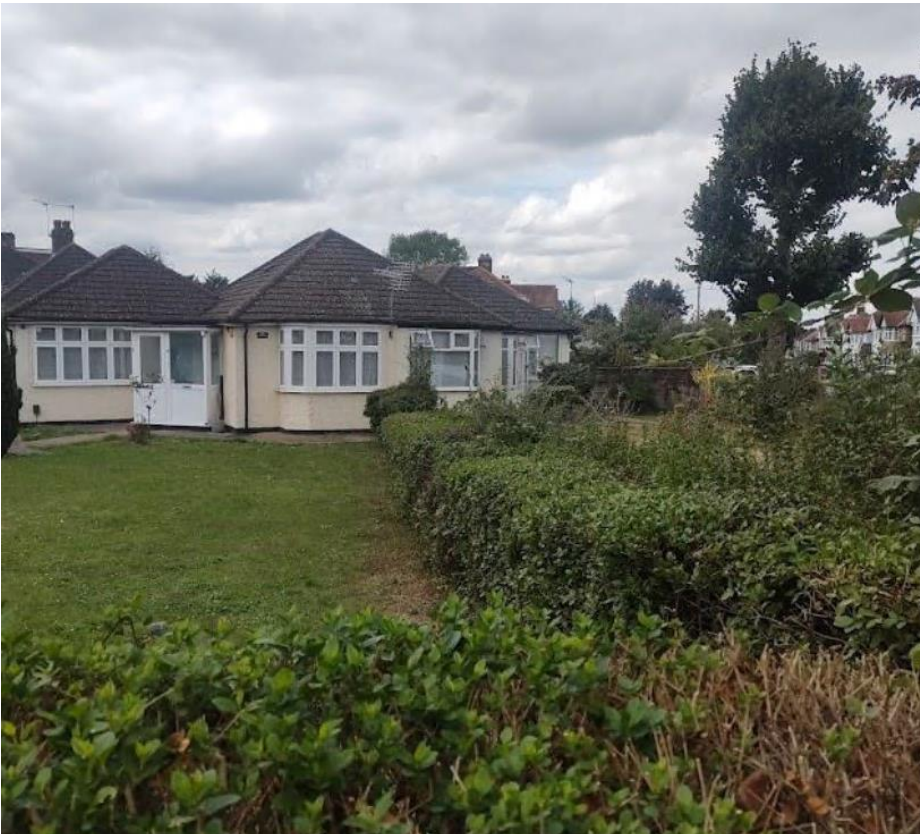
Front Elevation of 40A Somervell Road:
